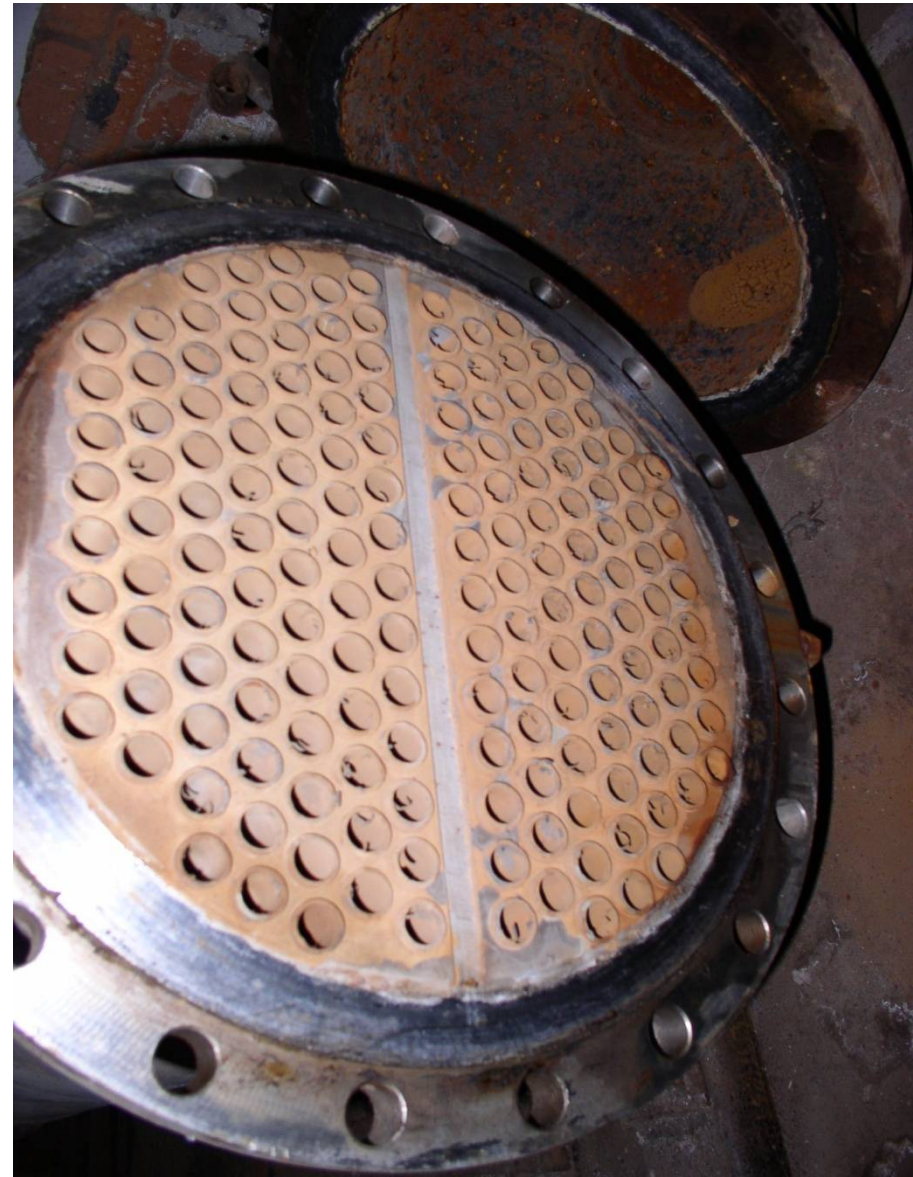
Examining the work of first RAU prototype protecting the steam heat exchangers for hot water on «Ilyich iron and steel works»
